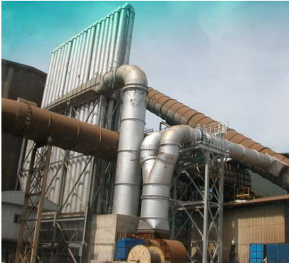
FABRICATION & INSTALLATION OF COOLER & DUCT FOR SCSC-2006
